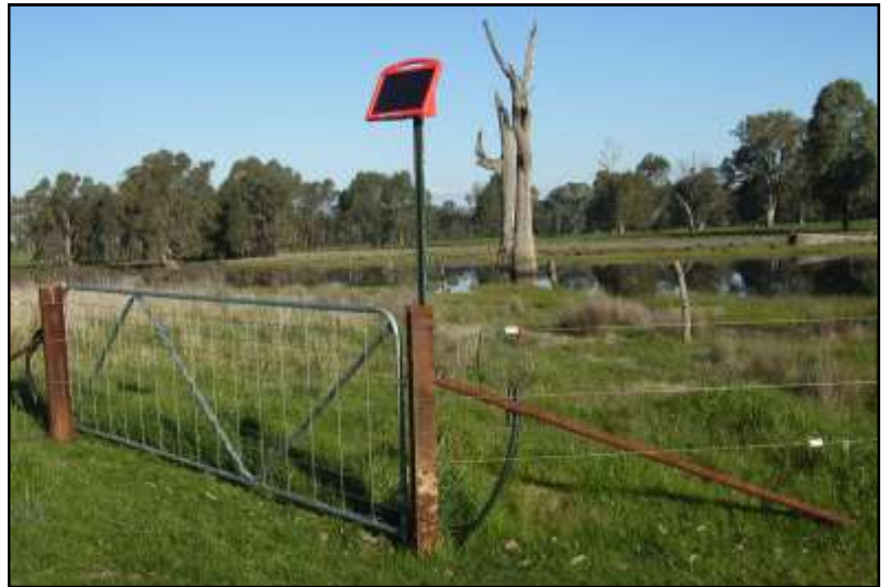
Photo 1: The fence protecting this wetland has been designed to be flood resistant. Very strong end assemblies of recycled railway iron support a minimal framework of three electrified plain wires powered by a stand-alone solar-powered energizer.
