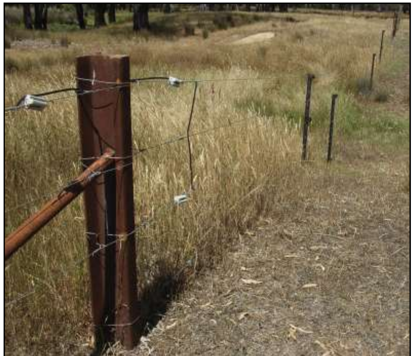
Photo 2: End assemblies are the most expensive part of a fence to install. A flood channel crosses this fence from left to right, & this length has been wired as a separate "sacrificial" section (note the end assemblies each side of the channel). Each section of the fence between the posts have been wired separately (note the wiring at the post in the foreground).
