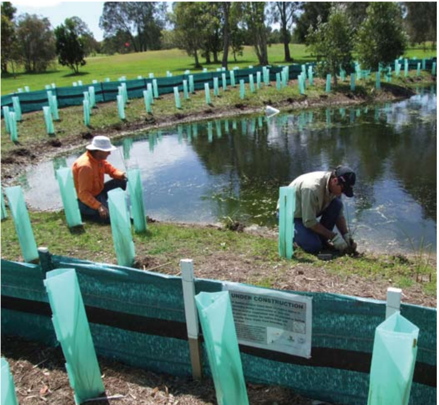
Consideration needs to be given to the protection of planted seedlings from damage by animals, mowers and climatic conditions (such as frost and drying winds). Photo Wendy Neilan
