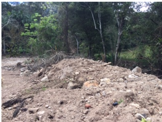
Shot showing bank after excavator work on water's edge
