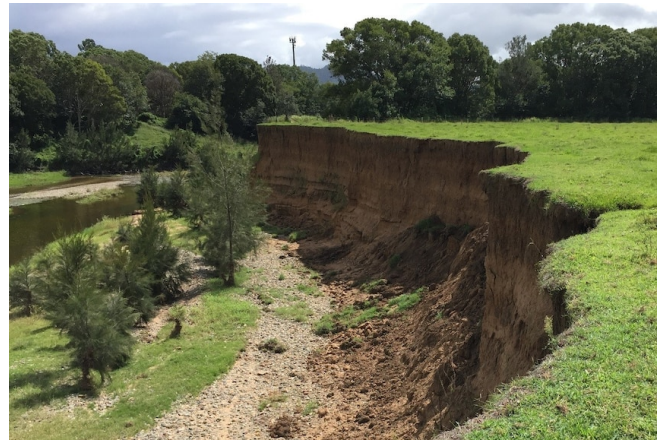
April 2019 before restoration
