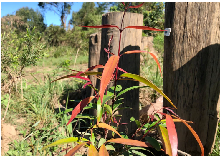
The piles have stopped erosion and plantings are thriving.
