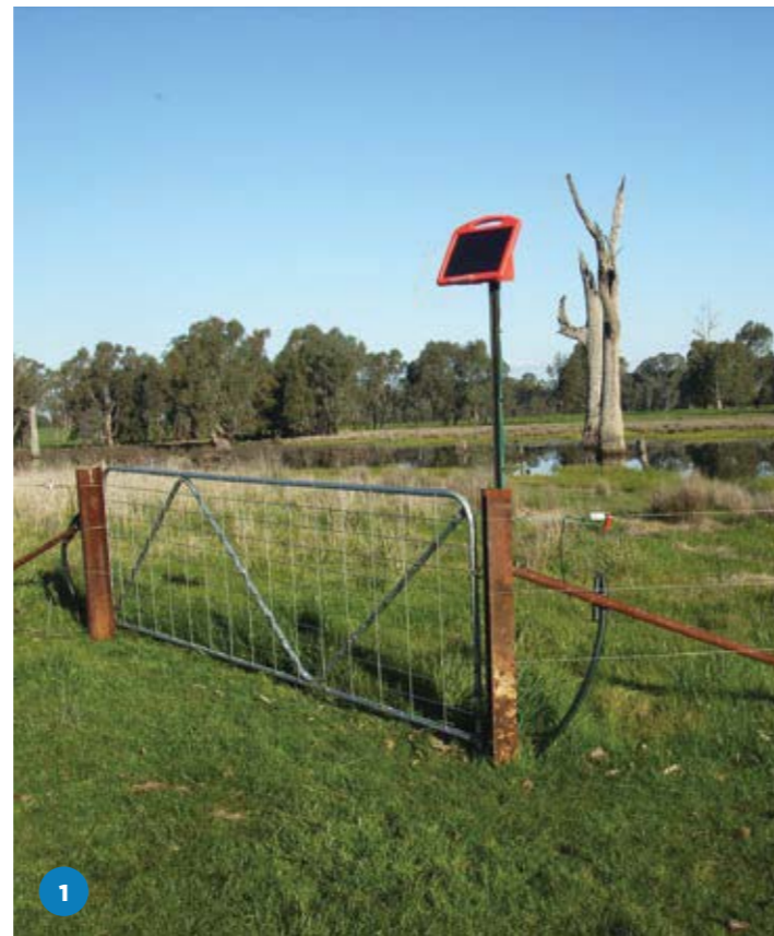
IMAGE 1: The fence protecting this wetland has been designed to be flood resistant. Very strong end assemblies of recycled railway iron support a minimal framework of three electrified plain wires powered by a stand-alone solar-powered energizer.
