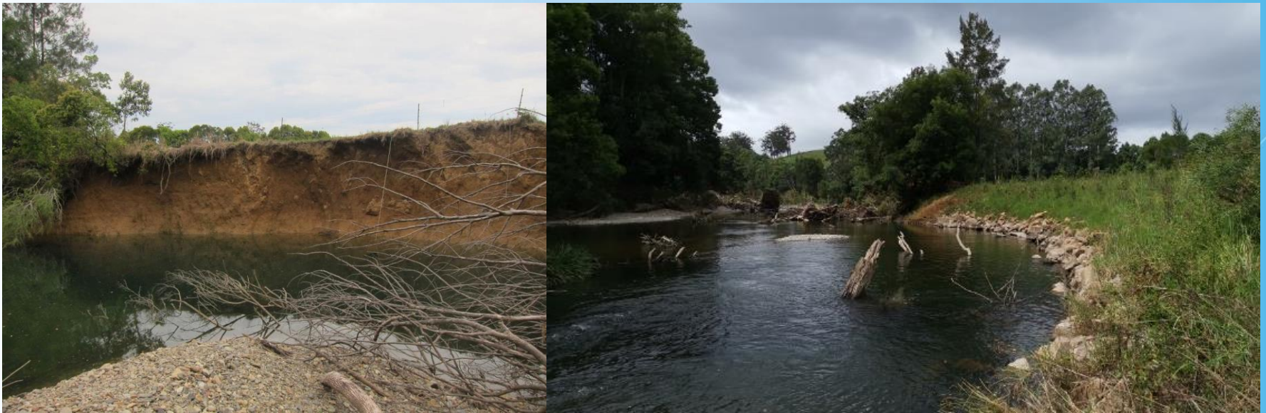
Composite logjam and bank battering Orara River
